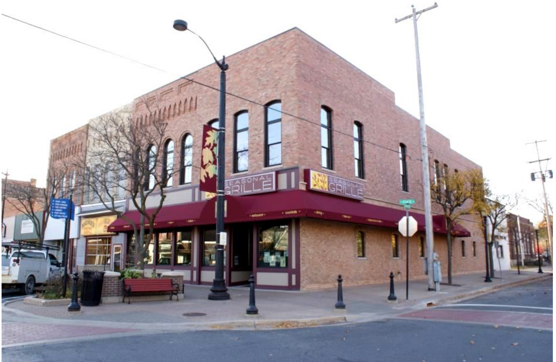
Exterior Building Restoration – AFTER
