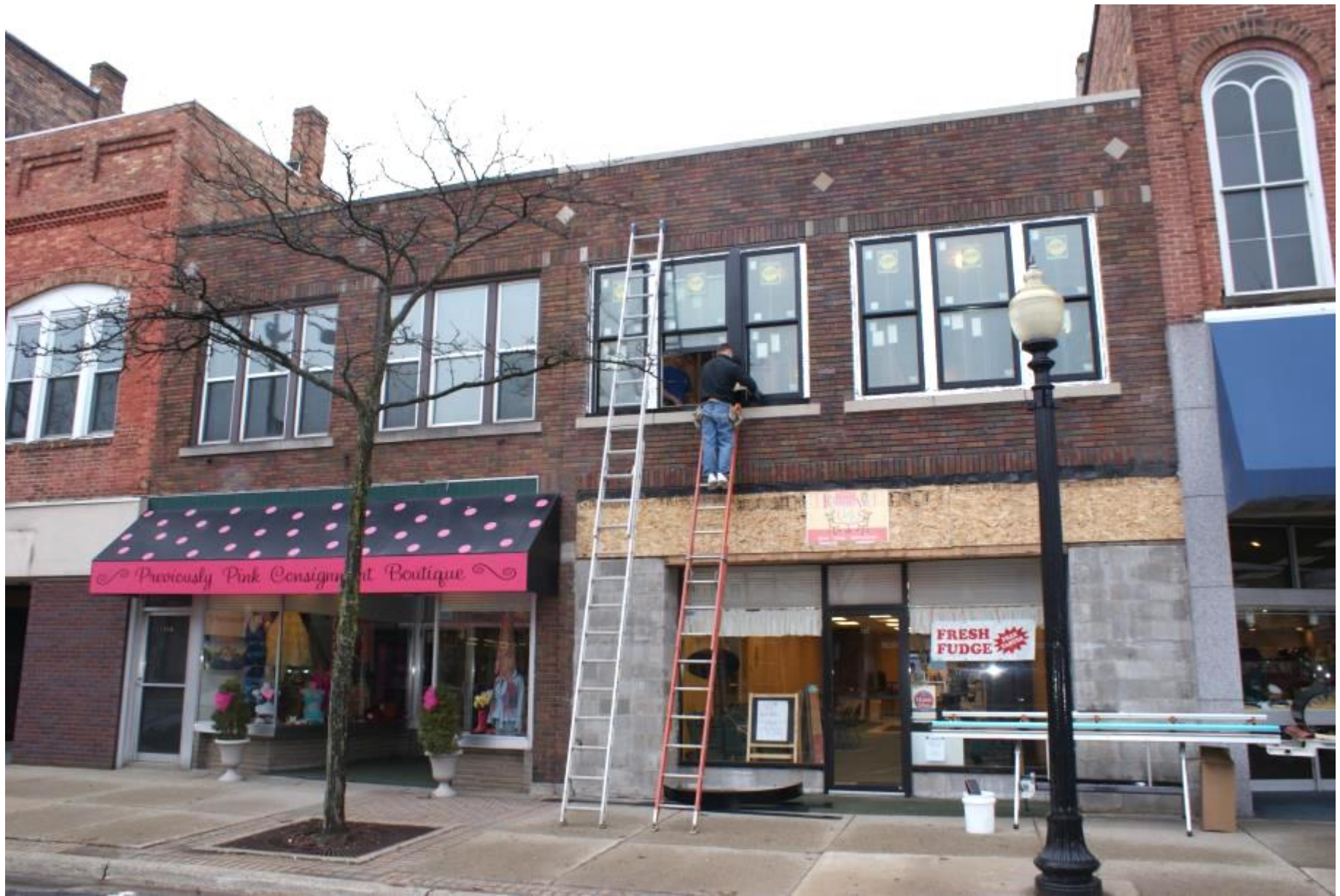
Exterior Building Restoration – AFTER
